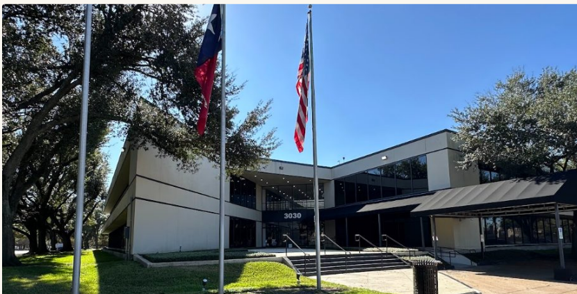
RECENT RENOVATION & FINISH-OUT WORK
